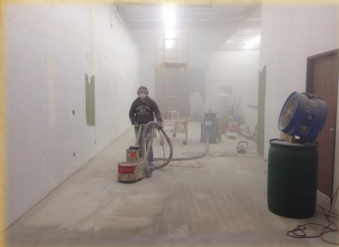
Prepping the Floor
